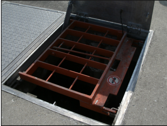
Figure 7-1 Palace Road PS – Safety Grate (Photograph)
