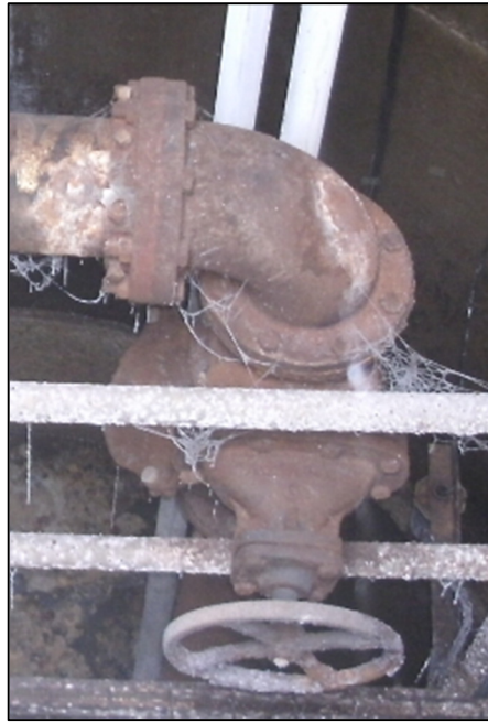
Figure 7-2 Kenwoods Circle PS – Isolation Valves (Two Photographs)
