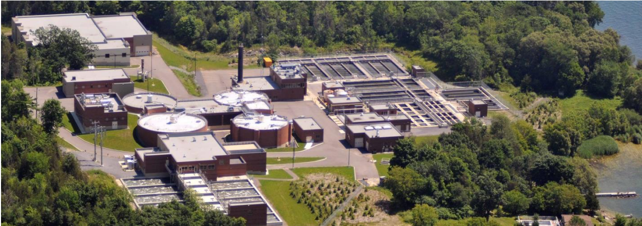
Figure 4 - Ravensview Wastewater Treatment Facility, Kingston, Ontario*
