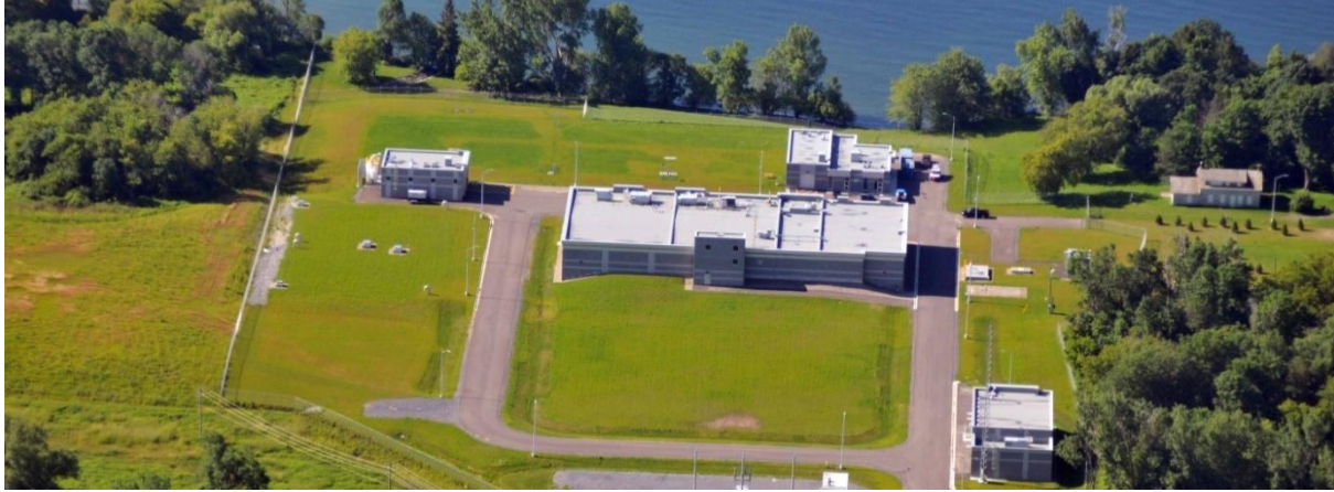
Figure 3 - Point Pleasant Water Treatment Plant, Kingston, Ontario*
