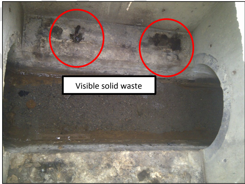
Figure 2: Visible Solid Waste in 17MH4
