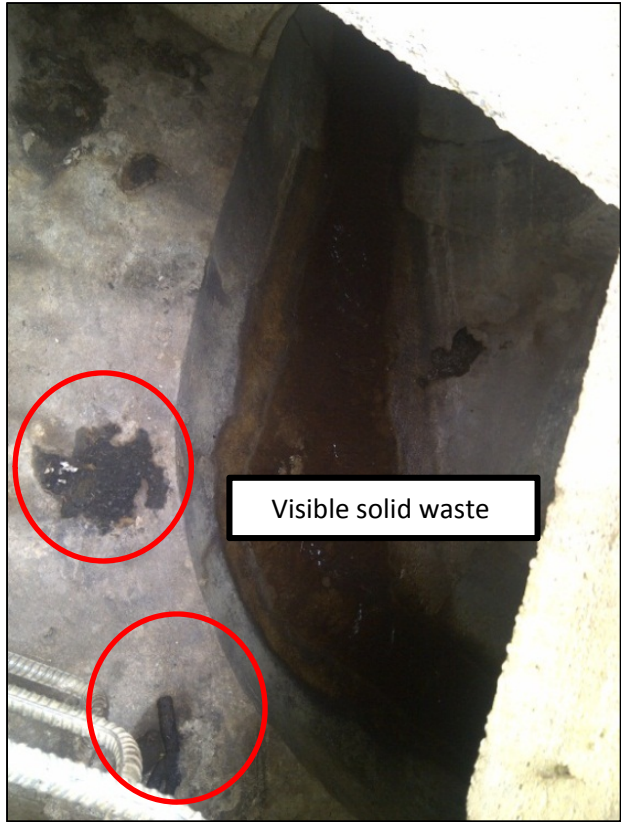
Figure 1: Visible Solid waste in 17MHC
