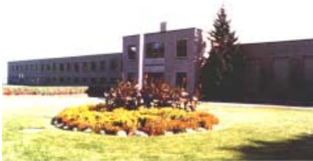
Water Treatment Plant 302 King St. West. Kingston, On. K7L-2X1 phone: 613-546-1181 ext. 2296 fax: 613-542-7096
