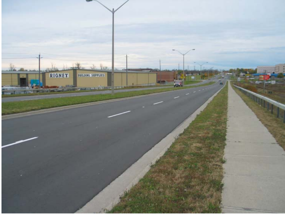
Plate 13. 1H: Sir John A. MacDonald Blvd south of overpass.
