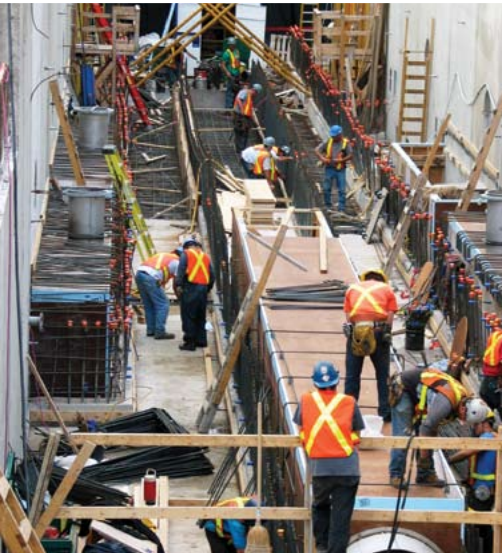
Forming the backwash channel at the base of the BAF.
