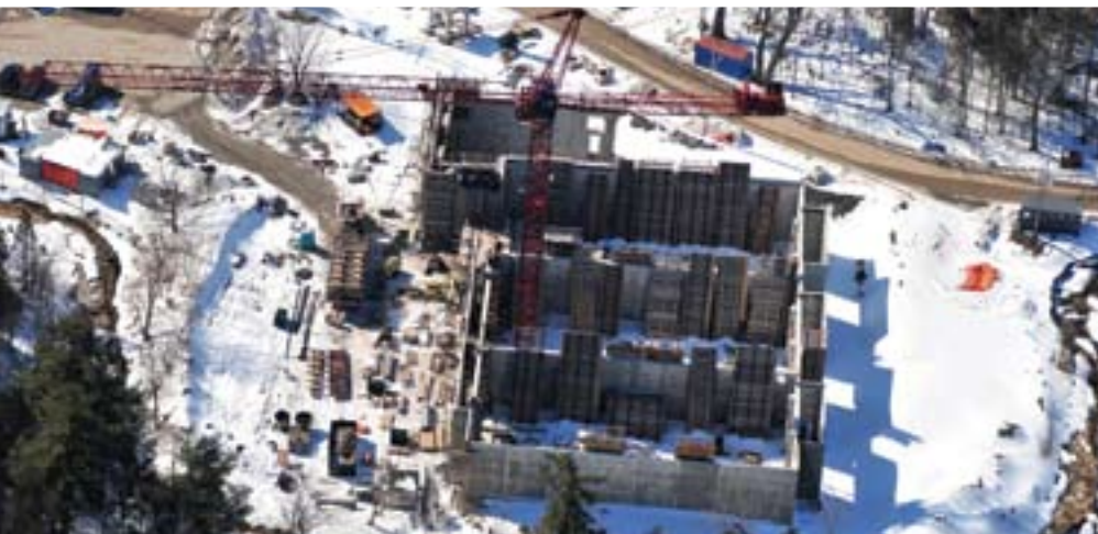
Aerial of the new three-cell biosolids storage building.
